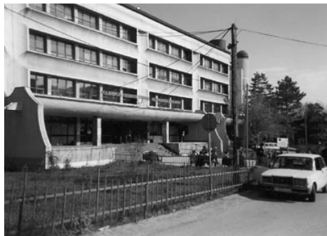
Obstetrics and gynecology hospital on the campus of the University of Pristina Medical School.
